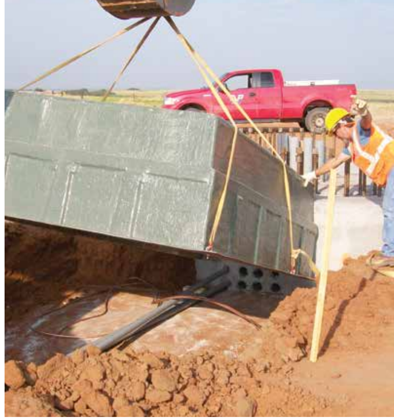
TOP: Setting transformer base on a wind farm project.
