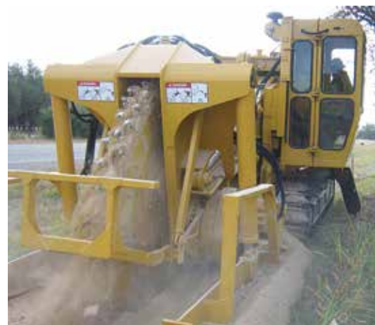
TOP RIGHT: Hydro Excavation Equipment. BELOW RIGHT: Rock Saw cutting limestone.
