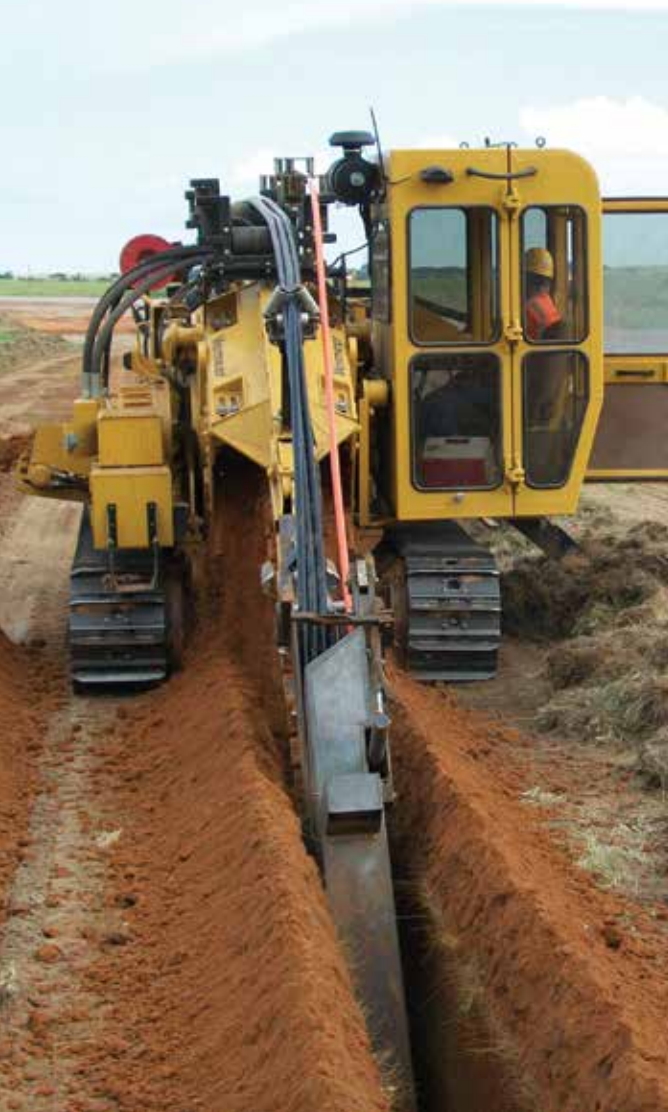
ABOVE LEFT: Trenching and placement of power cables and communications duct in a single pass.
