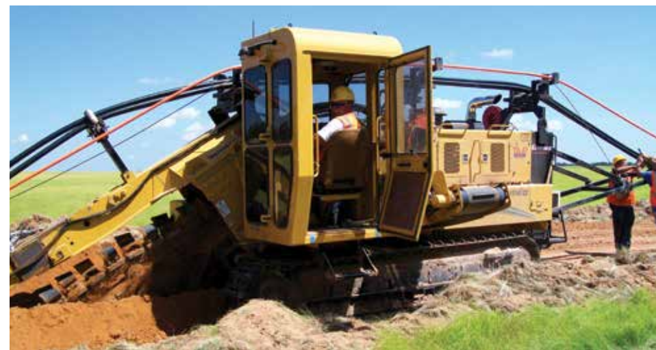
LEFT: Trenching on a wind farm.
